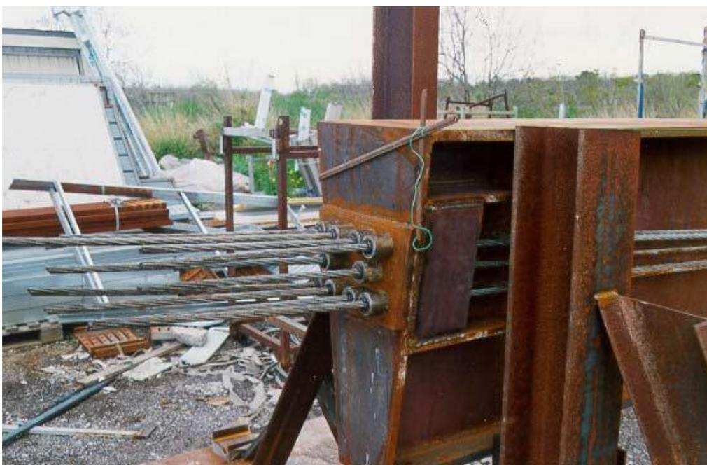
FIGURA 2-16 - DETALHE DAS ANCORAGENS EM UMA VIGA METÁLICA PROTENDIDA
